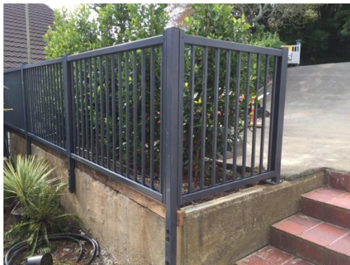
Figure 1. Moduline safety fence installed with fixings to a concrete retaining wall.
